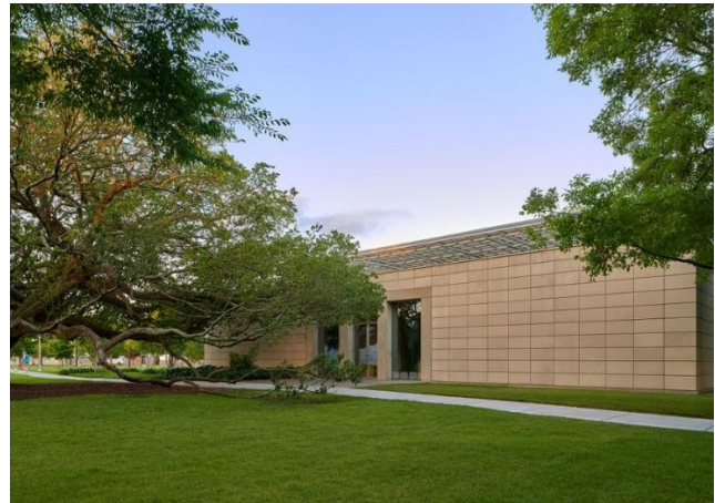
Exterior view of the Cy Twombly Gallery
